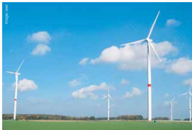
Renewable energy from the North: ewz wind turbines in Dörnte (Lower Saxony).
