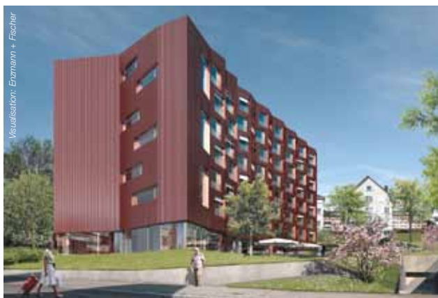
Compact building envelope, sun-facing windows, wood pellet heating: the Trotte Retirement Home
