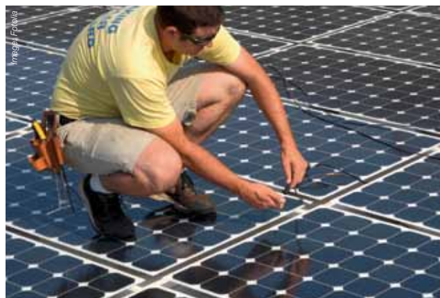
Solar energy, the growth industry: installation of a photovoltaic system.
